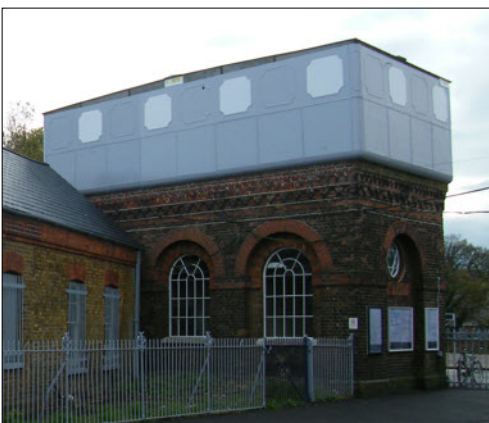
The 1863 water tower built of brown brick with red brick dressings. Note the elaborate modillion cornice and round-headed windows. This building is an excellent example of the high standard of bricklaying in the Victorian age. Note the bricked-in former doorcase below the bull's-eye window
