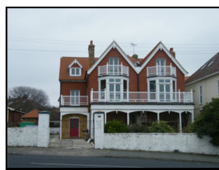
71 Sea Road, Westgate-on-Sea (Replacement of balconies, windows, etc)
