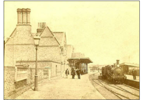
View inside Margate West with a London-bound train on Platform 2. This photograph dates from c.1900
