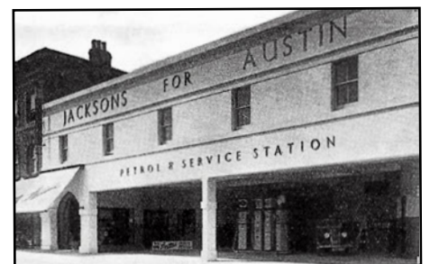
The new facade installed in 1937
