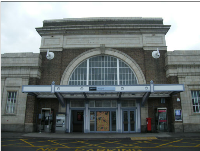
The entrance to Margate Railway Station today. Note the holders for flagpoles on either side of the entrance and the small lettering 'MARGATE' alongside the even smaller letters 'southeastern' on the front of the protruding shelter. Then compare that lettering with the former large lettering shown in the accompanying sepia photograph proudly announcing that the station was originally part of the Southern Railway
