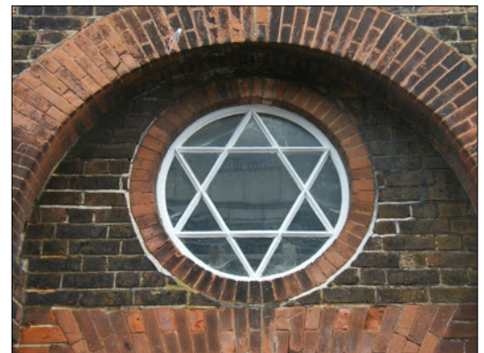
Close-up of the brick single ring bull's-eye window in the water tower. Note that the glazing bars are in the pattern of the Star of David
