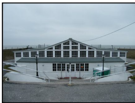
Westgate Pavilion, Westgate-on-Sea (Refurbishment)
