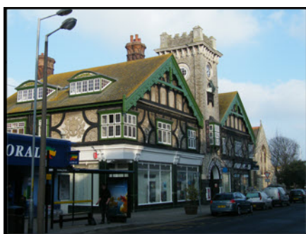
Town Hall Buildings, St Mildred's Road, Westgate-on-Sea (Refurbishment)
